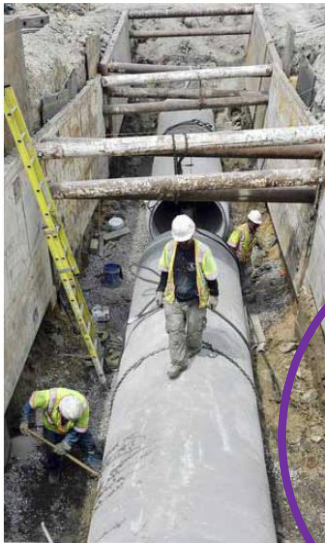
Baltimore Water Pipe
